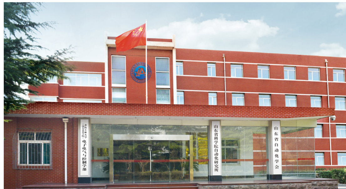
山东省科学院自动化研究所大楼 Institute of Automation Building, Shandong Academy of Sciences
